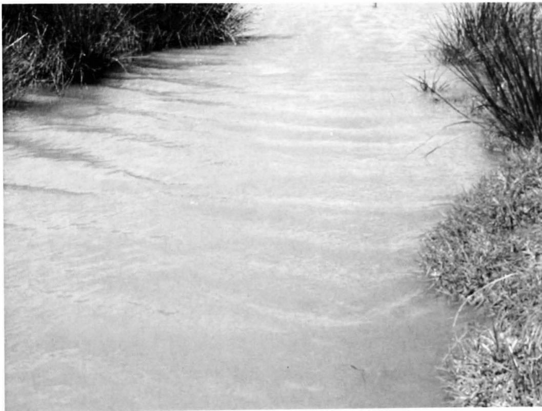
Figure 8.4: One of the three settlement lagoons showing orange colouration of acidic and polluted mine water (with ochre precipitate) that has passed through the PRB at Shilbottle site. This highly turbid orange water contains solid iron oxyhydroxide; the wetland effectively removed these solids.
