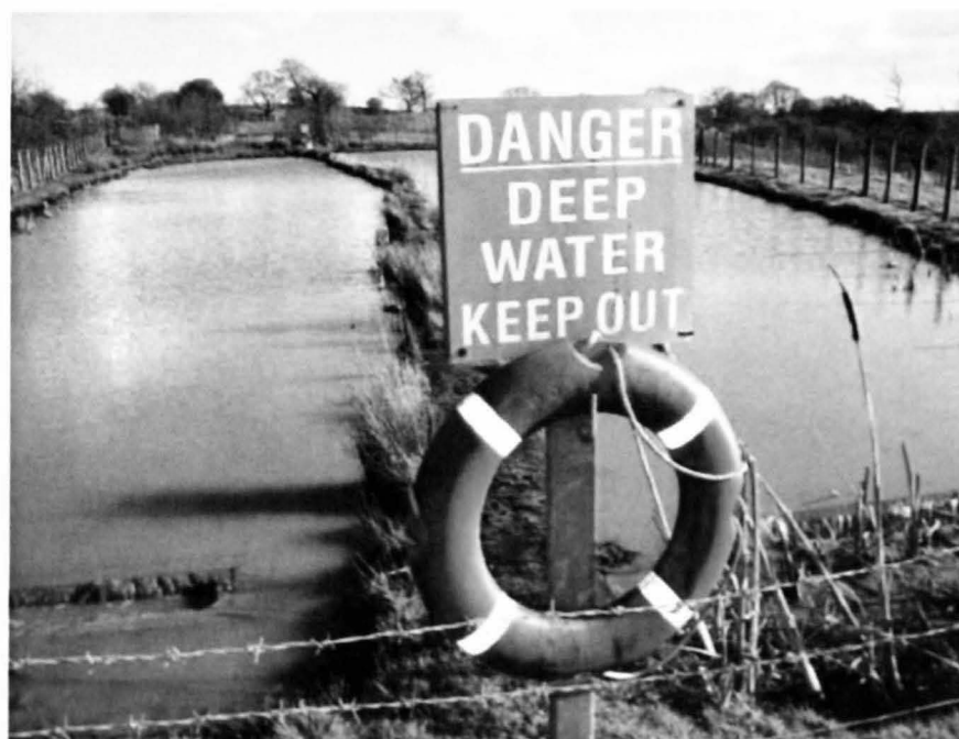
Figure 9.2: Photograph taken September 26, 2006 by Kola, showing two parallel settling ponds where ochre precipitation takes place after pumped water from the drift has been aerated through cascade.
